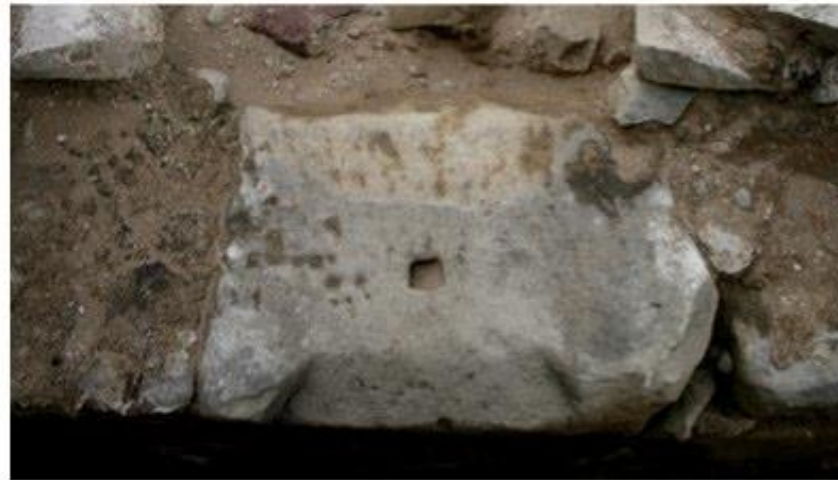
The window sill showing the stanchion hole and carved splay.
